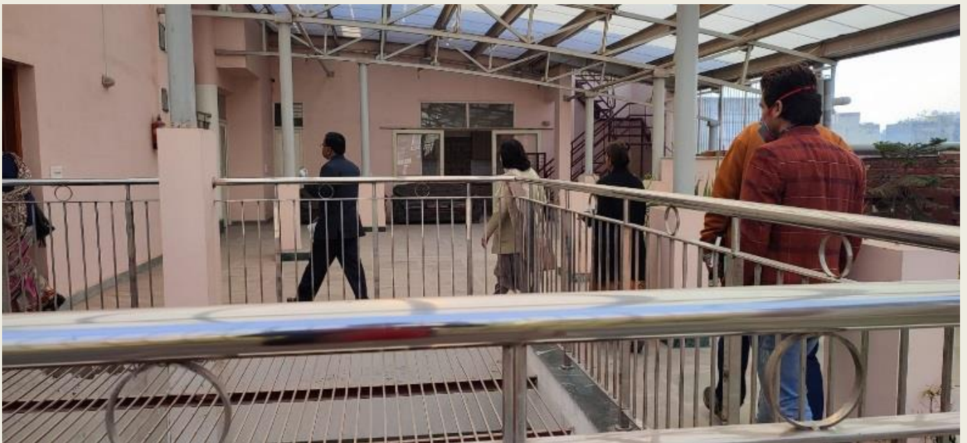
Inspection of the ramp around the building
