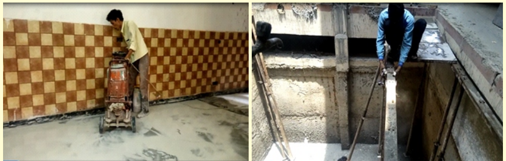
Construction of ASRA Special School
