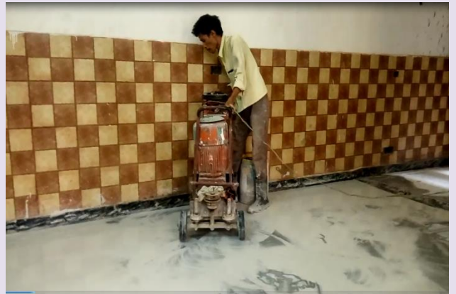
Construction of ASRA Special School
