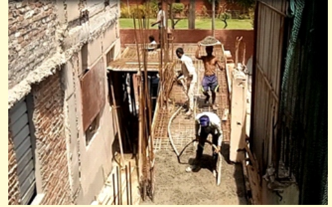
Construction of ASRA Special School
