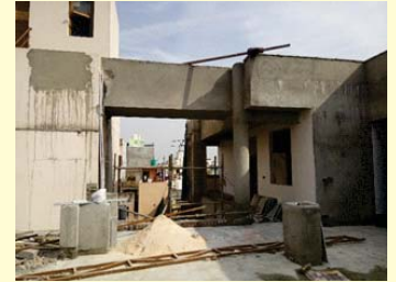
Construction of ASRA Special School
